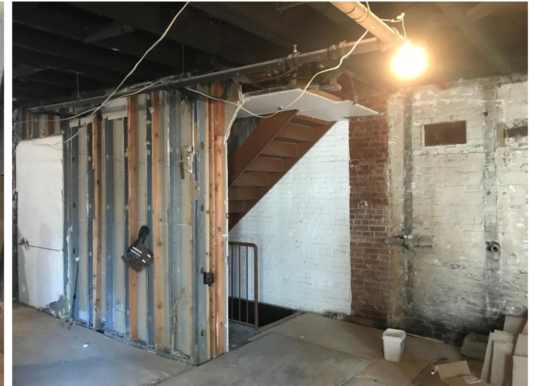
Existing wall was removed for new steel beam on 3rd floor
