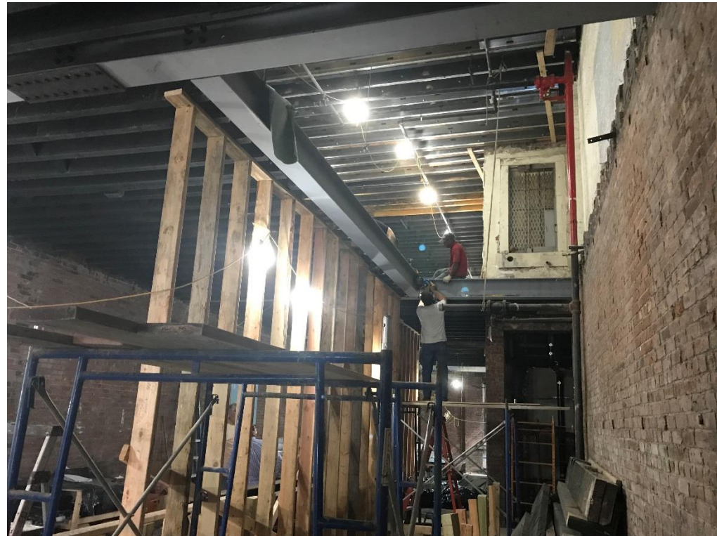
New steel beam was installed on 2nd floor
